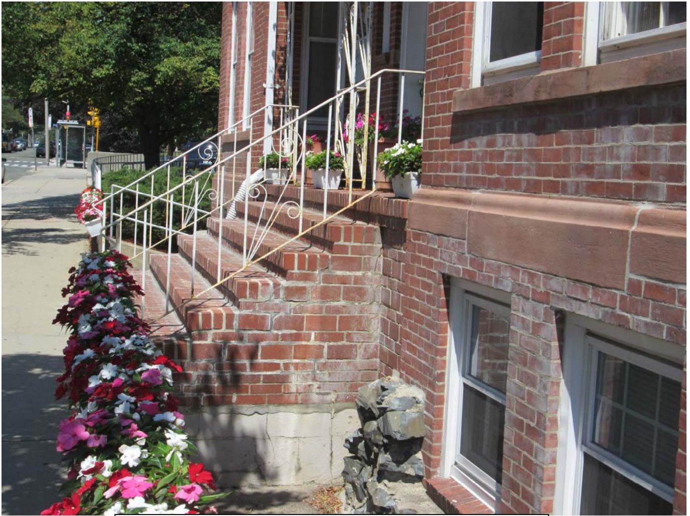
17-19 Highland Avenue showing the fracture patterns of the bricks after repointing.
